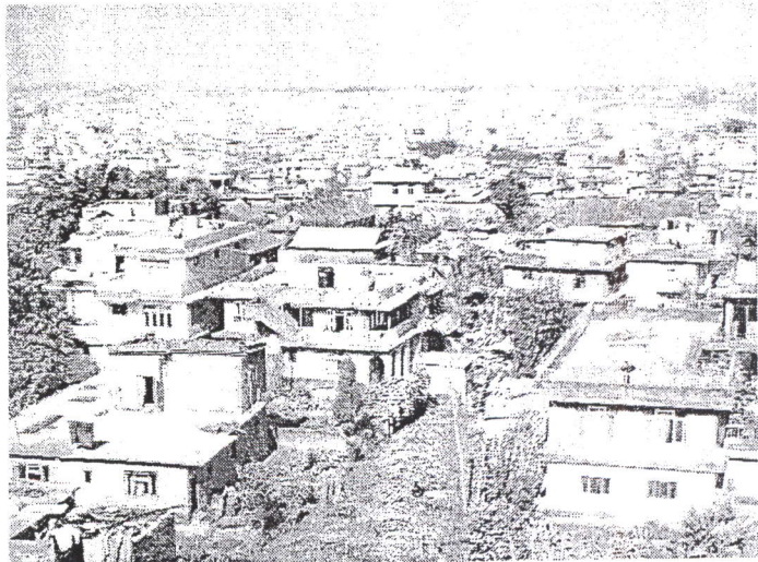
Fig. 4.2 Buildings are mushrooming in Sunakothi Case study area.
