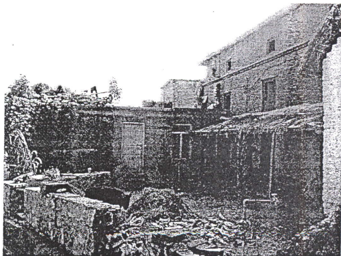
Figure 4.13. Traditional building standing at roadside. (Saibu Land Pooling Area)
