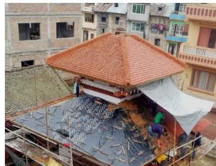
Figure 87 Different jhingati tiles and plastic waterproof layer used on roof in the reconstruction
