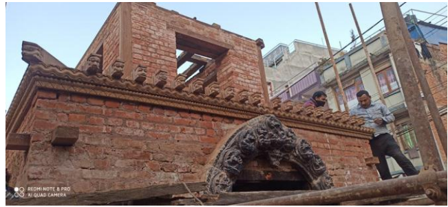
Figure 70 stone toran above the entrance
