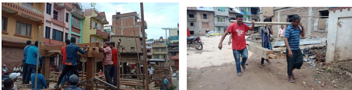
Figure 65 Local people helping out in the construction work
