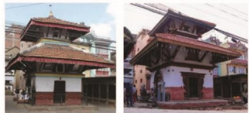
Figure 2: Mahalaxmi temple before and reconstruction
