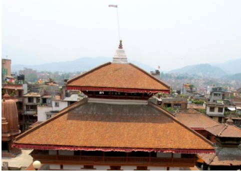
Figure 16 Pinnacle on the second floor roof
