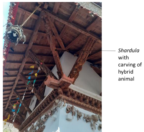
Figure 93 struts south eastern corner lower roof new
