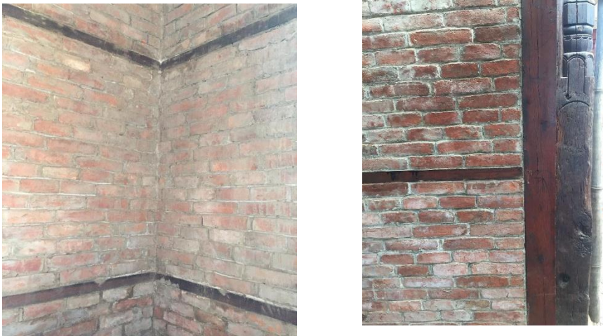
Figure 25 Corner post first floor
