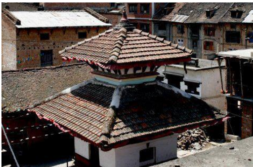
Figure 87 Different jhingati tiles and plastic waterproof layer used on roof in the reconstruction
