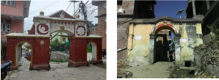
Figure 30 Northern gate (left) and eastern gate (right)
