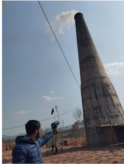
Measurement of surface temperature
