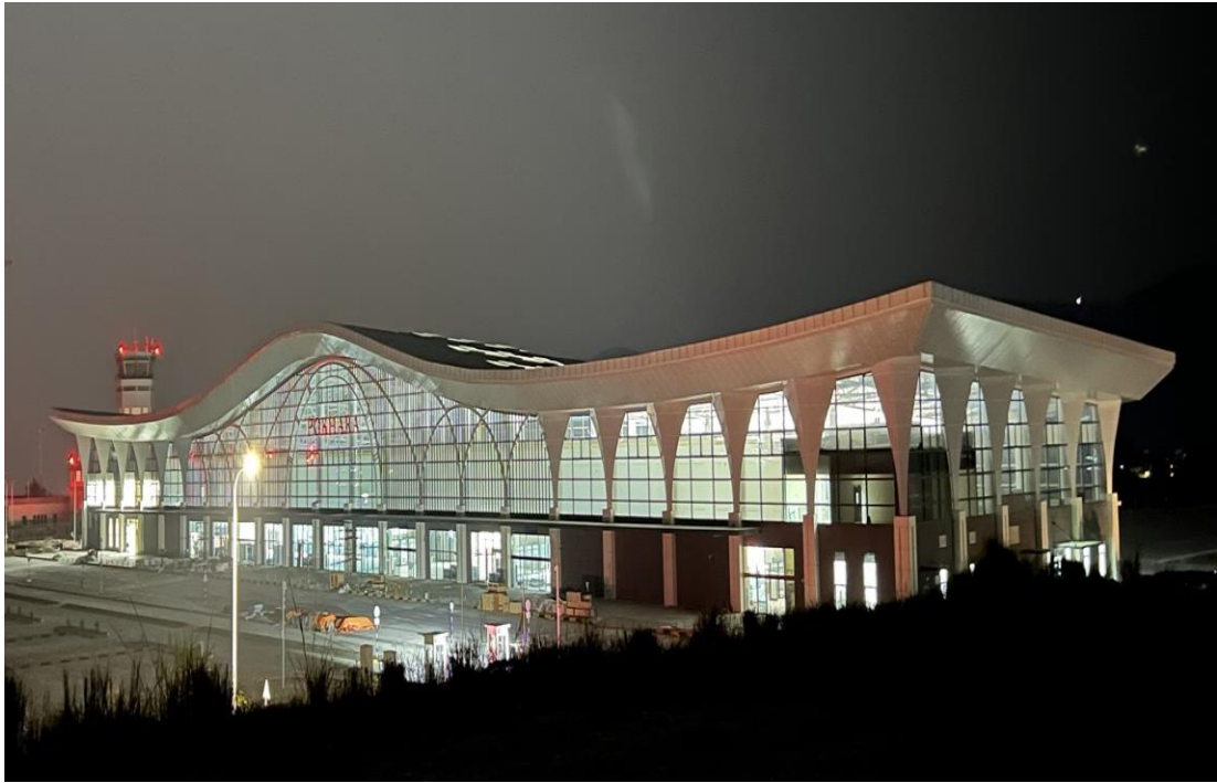
Figure 1.1: Night view of Terminal Building of Pokhara International Airport
