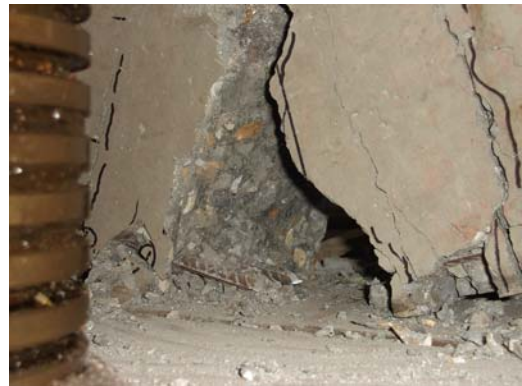
Photo 24: Main Bar Ruptured in Beam C-T-1
