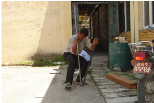
Photo 5: Rebar Fabrication
