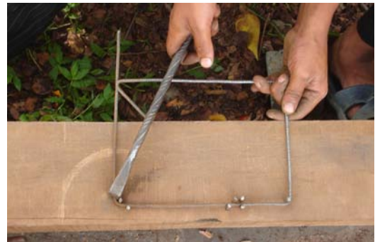
Photo 6: Shear Rebar Fabrication
