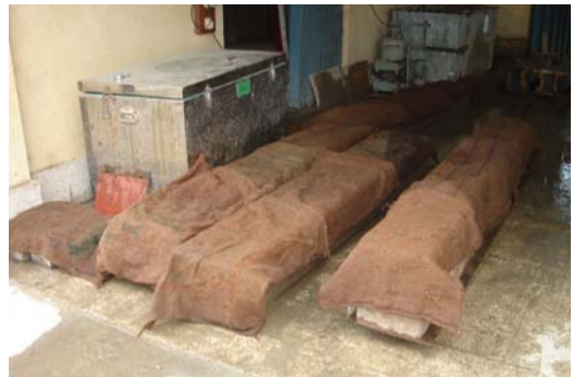
Photo 12: Curing Beam and Cubes
