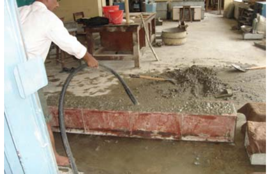
Photo 10: Concrete Vibration
