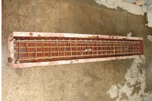
Photo 9: Rebar in the Form
