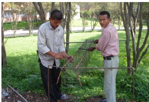
Photo 7: Rebar Fabrication
