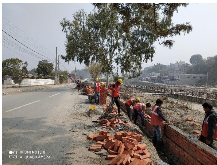
Figure 5-35 Ongoing Construction Works in Bagmati Corridor
