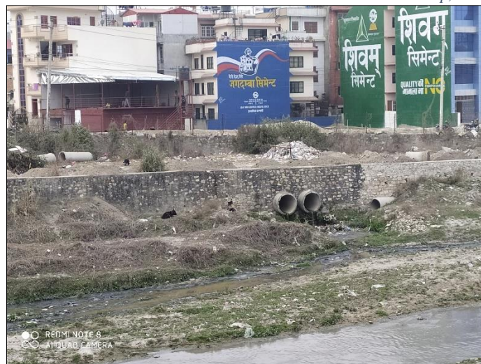
Figure 5-37 Disposal of Wastewater into Manohara River
