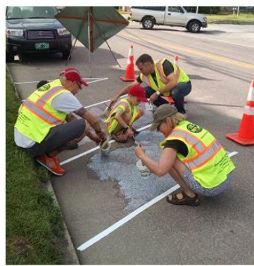
Figure 14: Pine Street, Burlington, VT (Street Plans)
