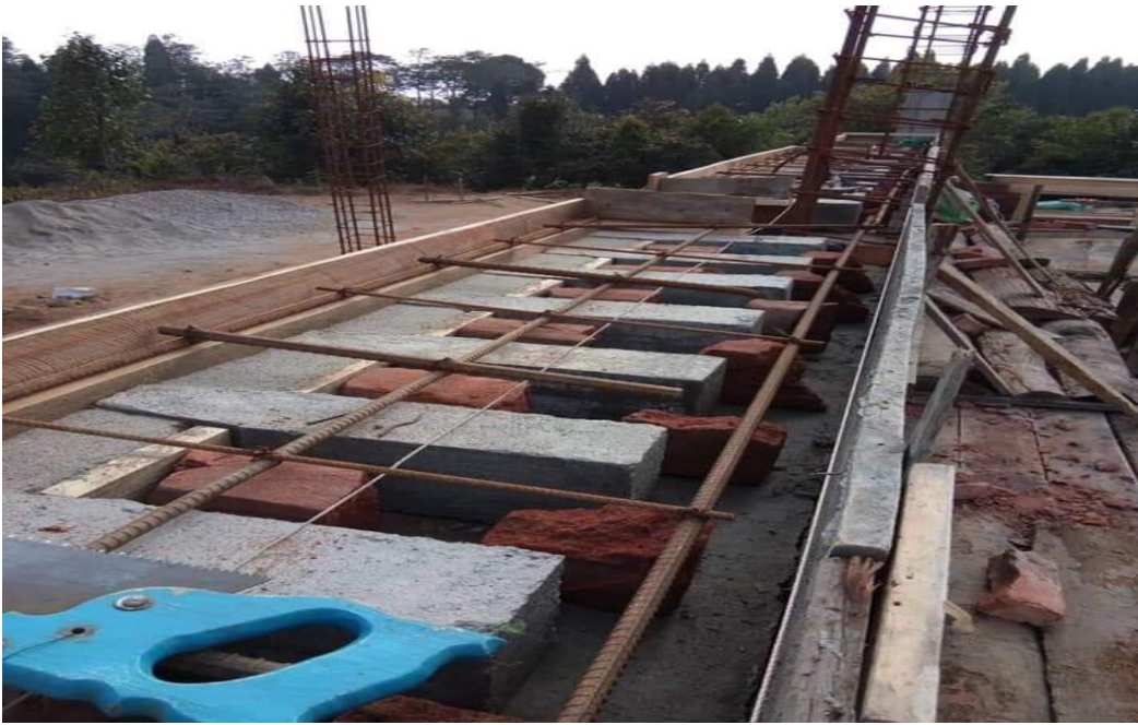
Fig. 16: gonpa foundation being constructed after 2015 earthquake
