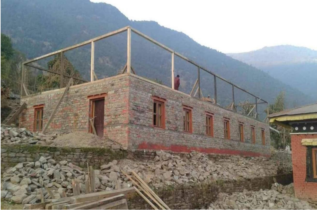
Fig. 20: Construction of monk quarters
