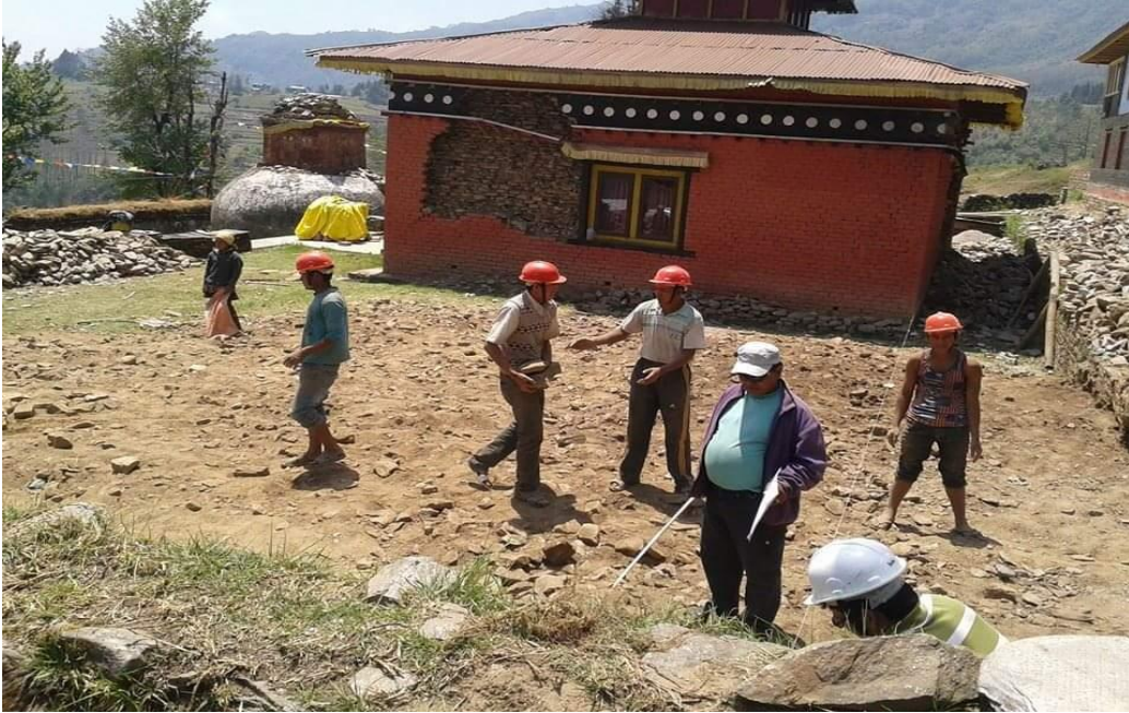
Fig. 26: damage on exterior wall by 2015 earthquake
