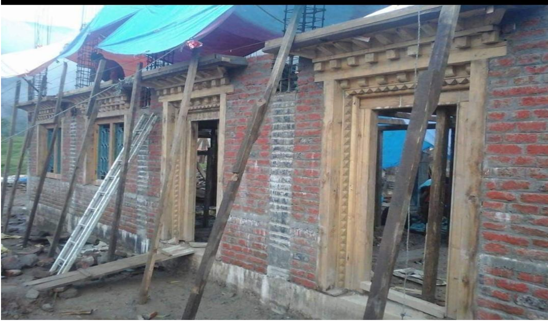
Fig. 22: Gonpa construction going on southern sides with two extra doors beside main altar door
