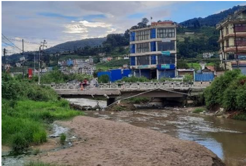
Figure 25: Present Condition of Pulbazar Bridge
