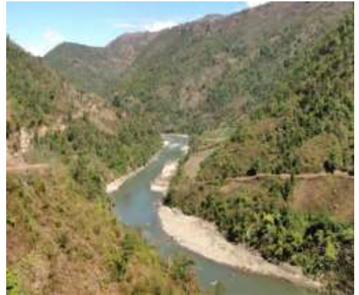
Proposed Dam Site of Budhigandaki HEP
