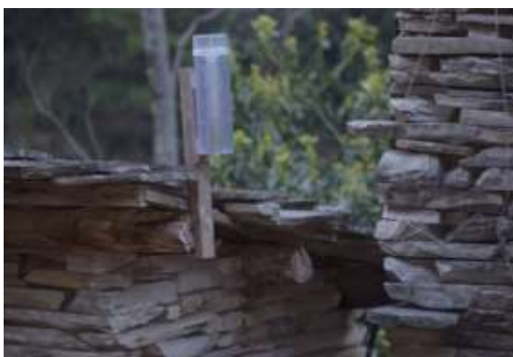
Rainfall Station at Salleri (Installed in 2020)
