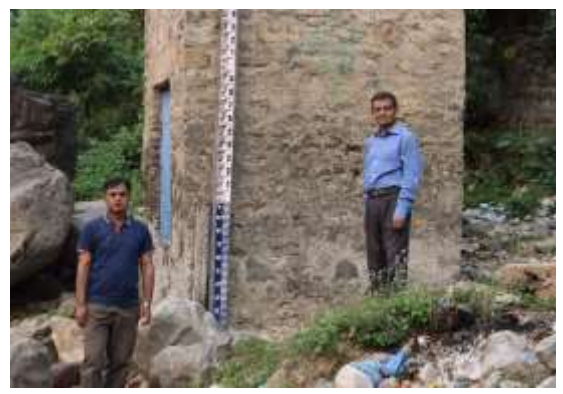
Gauge House of Budhigandaki River at Arughat (Station no. 445)
