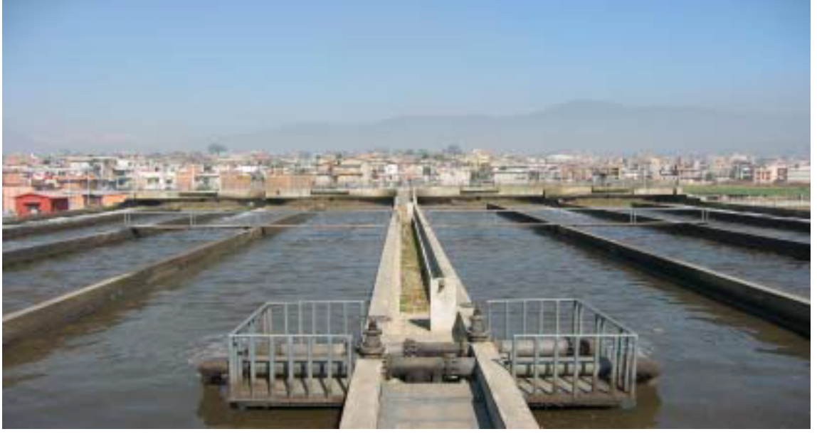
Figure 2.1: Guheshwori Wastewater Treatment Plant
