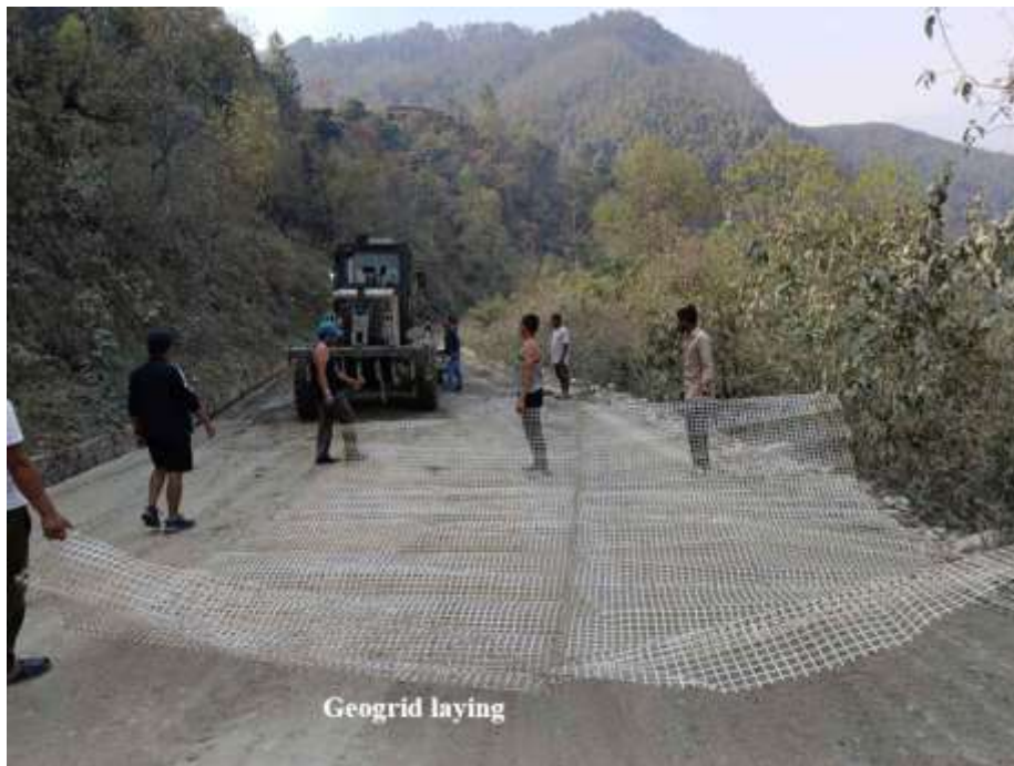
Figure 3.6 Placement of 40/40Q Biaxial Polypropylene Geogrid (Tensar)
