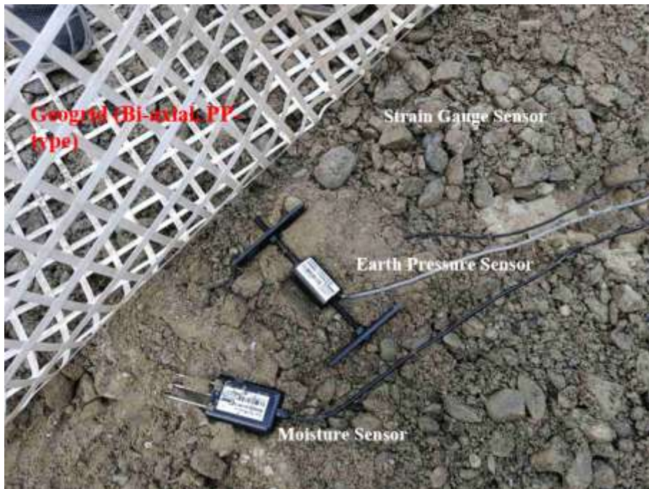
Figure 3.7 Placement of Sensors beneath Geogrid at Mid-Depth of Base Course
