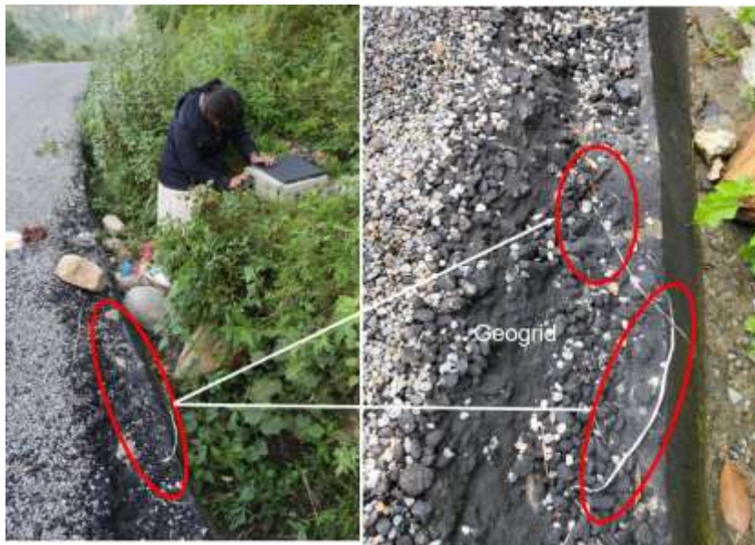
Figure 3.8 Data Logging at CH 1+800—Testing Setup (Left) and Geogrid (Right)
