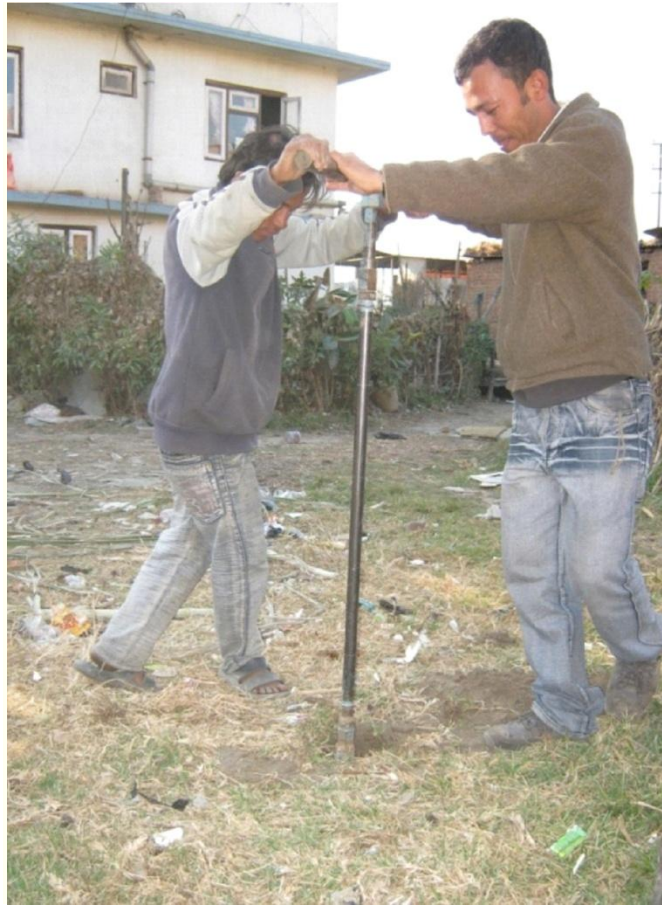
Fig. 3.3: Performing Hand Augering at Ekantakuna, in front of Sajha Yatayat Bhawan
