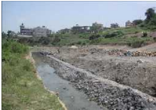
Figure 10.1: Bank encroachment and channelization for settlement
