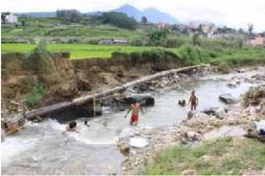
Figure 9.4: Scour of the river near water intake site at Nakhu Bazar
