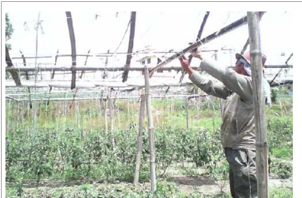
Construction Tunnel for Vegetable
