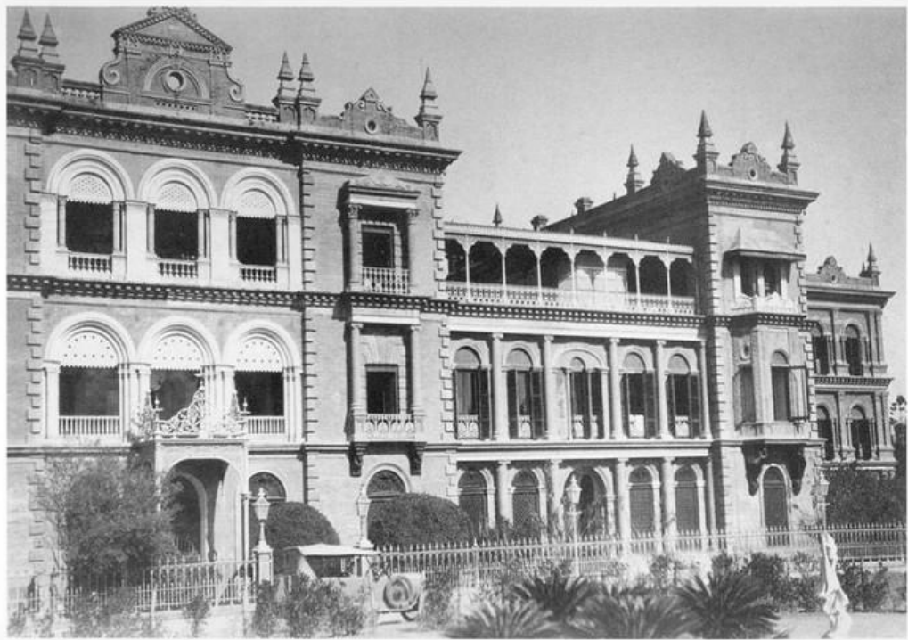
Lal Durbar before the earthquake. It was built for Bhim Shumshere in 1890, and at the time was one of the largest Rana palaces. Its brickwork led to its being called the Red Palace. In 1923 its northern wing was destroyed by fire, and the earthquake caused further damage. Today a part is incorporated into the Hotel Yak and Yeti.
