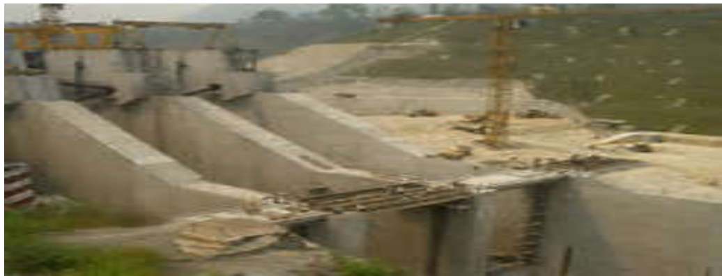
Construction and repairing of the canals (2004)
