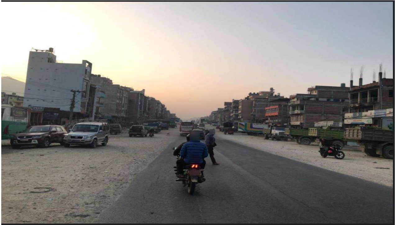
Figure 1.3.2 Existing Condition of the project Highway Section
