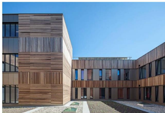
Figure H-6. Roof terrace.
