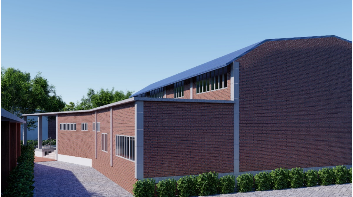
Figure 54 view of multipurpose hall
