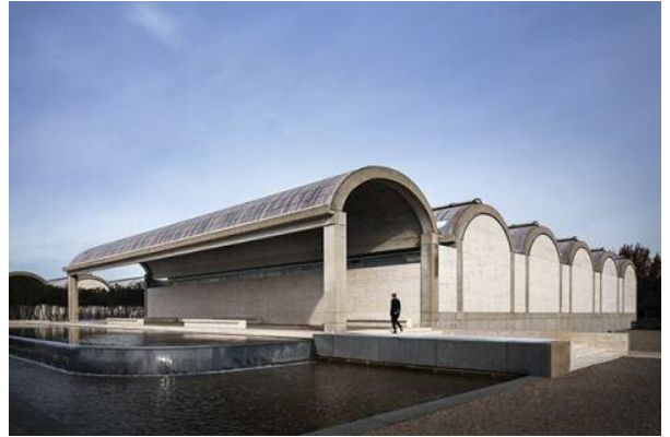
Figure 89: : Exterior of the building
