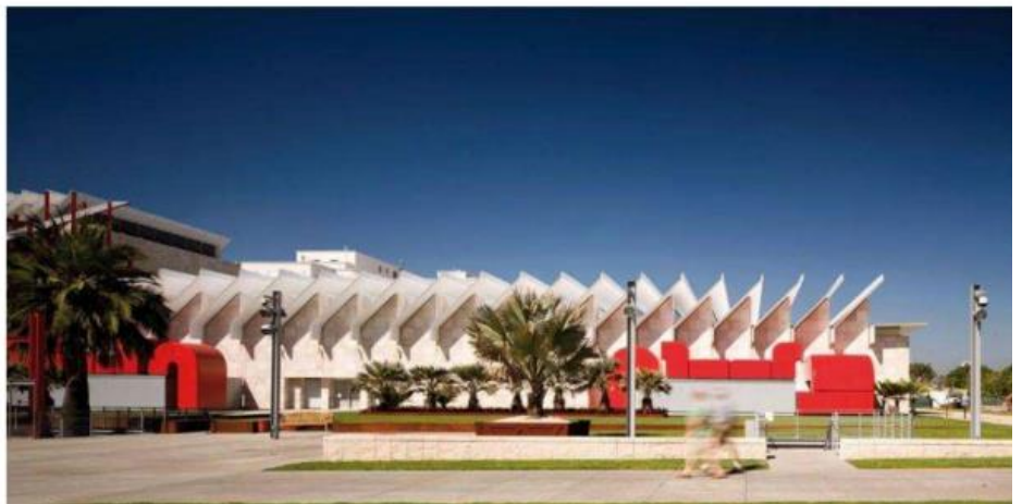
Figure 81: Resnick pavillion by Nic Lehoux
