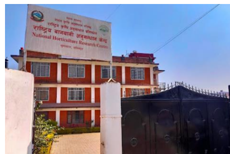
Figure 3.20- Horticulture Division building
