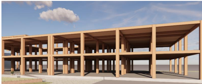
Figure 8. 5- Glulam and CLT structure
