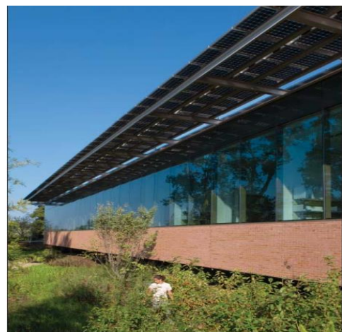
Figure 3. 42- Solar panels as shading device
