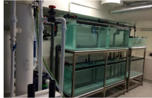
Figure 2. 29: Quarantine Tanks, source: aquariumtechnology.com
