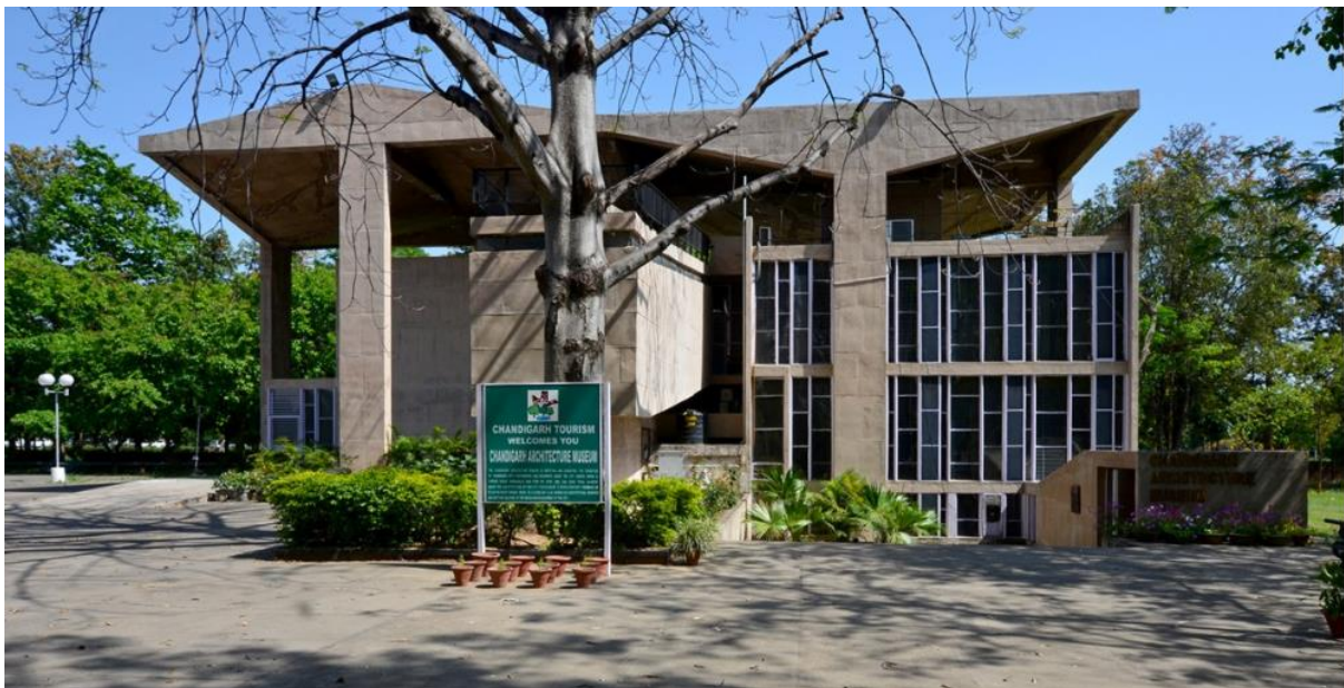
Figure 120 Exposed concrete exterior
