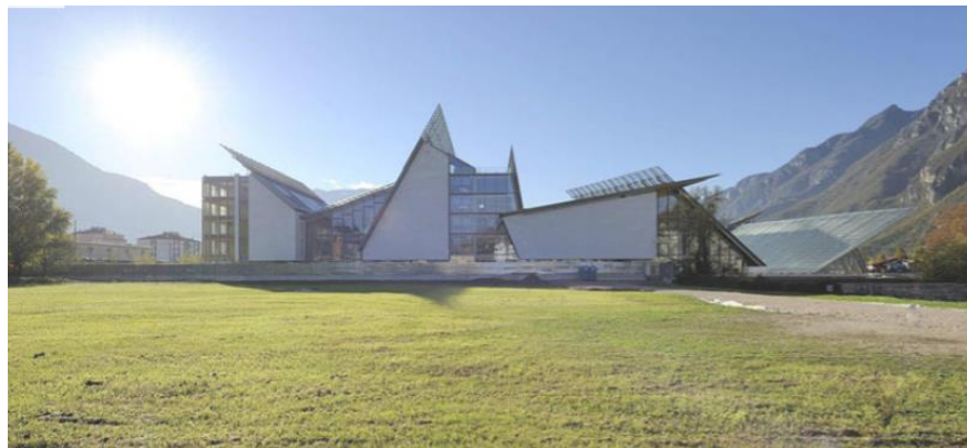
Figure 108 Roof uniting with background hill
