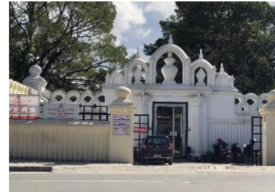
Figure 73 Main entry gate
