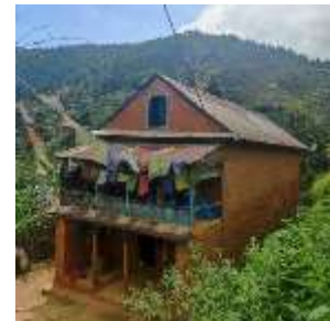
Figure 45: vernacular architecture of site
