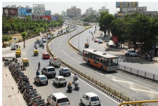
Figure 2.7: BRTS System in Ahmedabad
