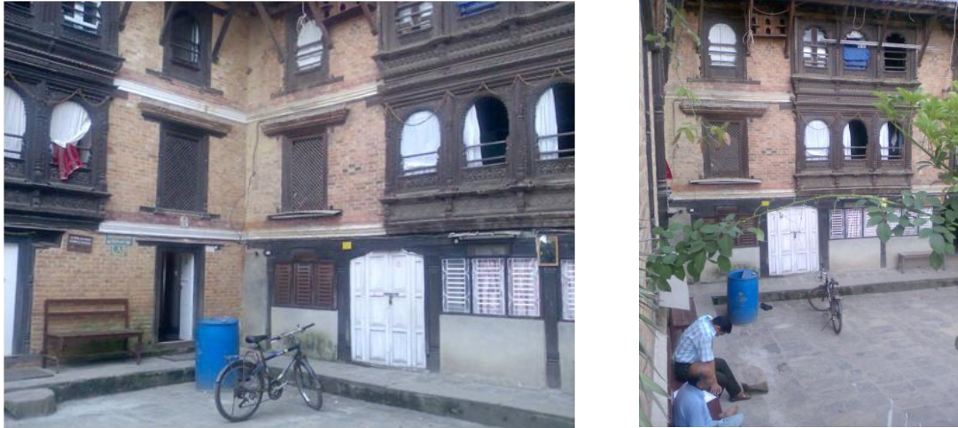
Fig. 2.7 A traditional house of private residential square ( Chukachhen ) in Patan
