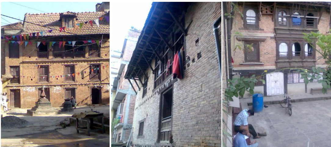
Fig. 2.3 Views of traditional residential buildings of Kathmandu valley
