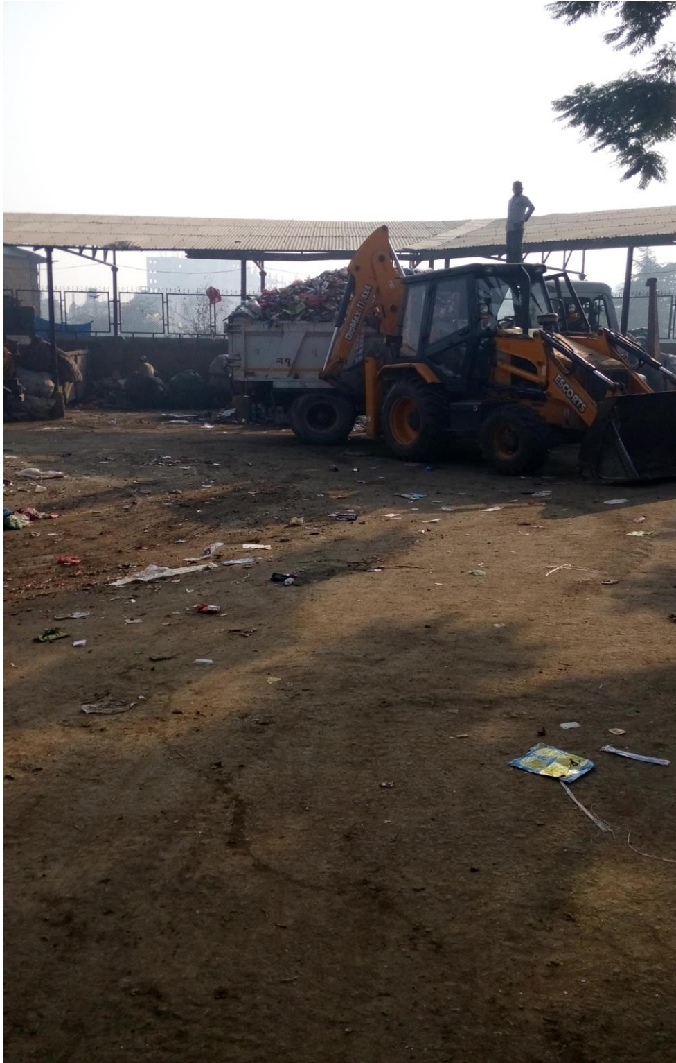
Ready to transport to the landfill site, Sisdole
