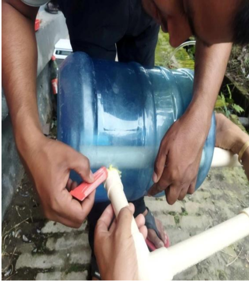
Figure: Fabrication of digester
