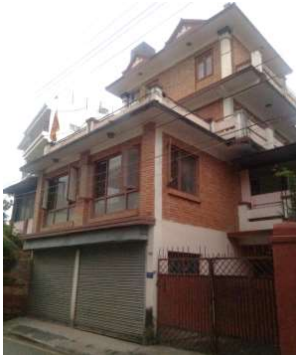
Figure 57: Investigated office building-6 (Civil Informatics and Solutions)
