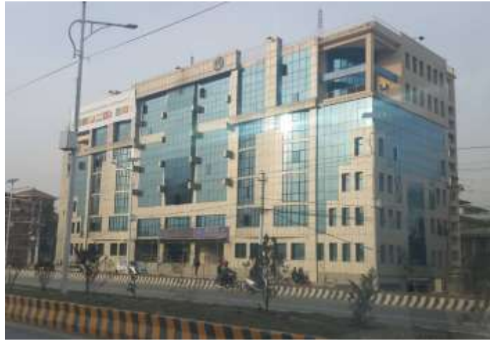
Figure 15: Office building-1 (Nepal Telecom located at Babarmahal)
