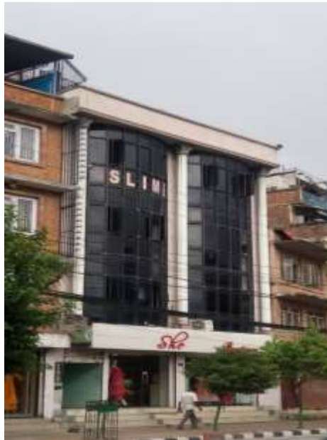
Figure 33: Office building-3 (AKG Associates Chartered Accountants)
