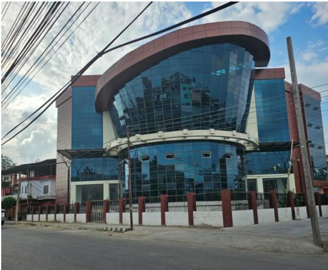
Figure 26: New Haat Bazaar building
