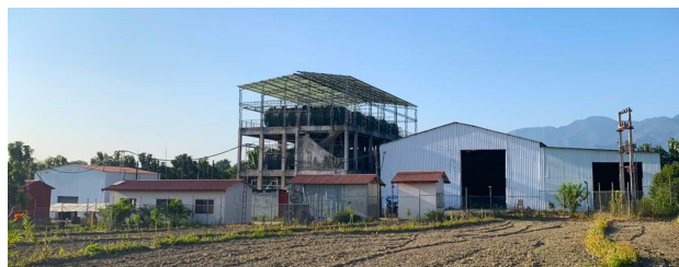
Figure 22: Venture WtE plant Pvt. Ltd.
