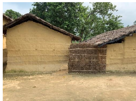
Figure 67: Houses with thatched roof in Matiyani Tole
