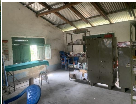
Figure 102: Inside of health centre in Tangiya Basti
