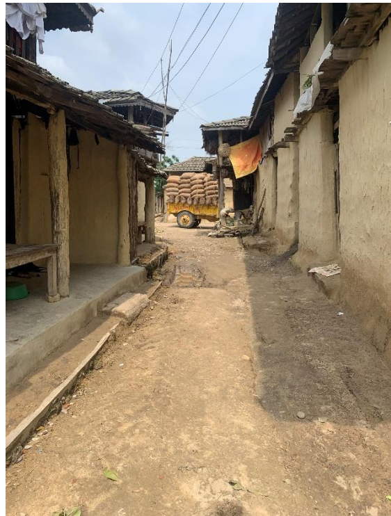
Figure 36: Internal Surveyed Road in Kathgaon
