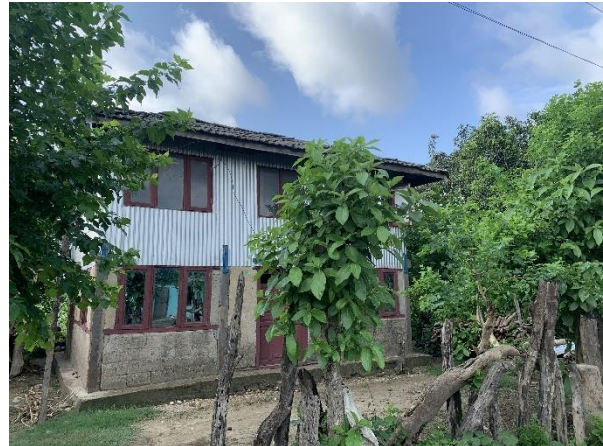
Figure 63: Stone blocks in Cement mortar
