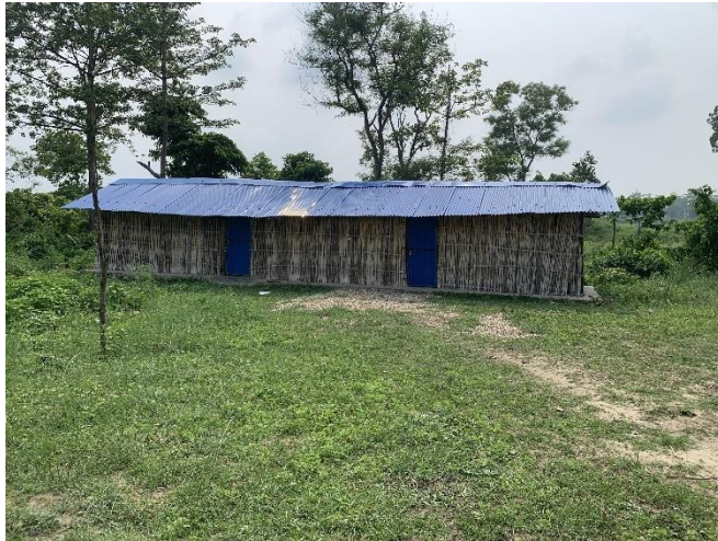
Figure 97: Shree Dalit Primary School
