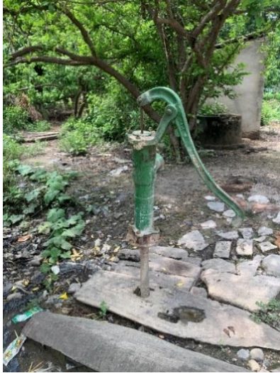
Figure 57: Tube well in Kath Gaon
