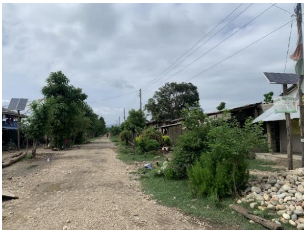
Figure 60: Solar Panels in Tangiya Basti
