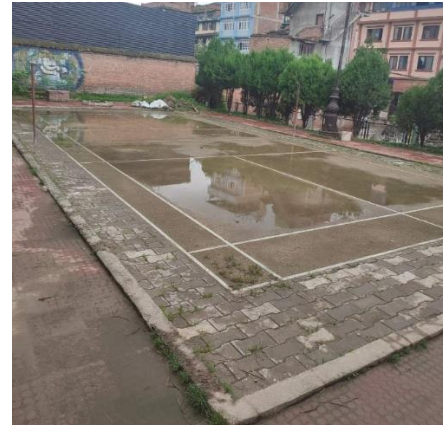
Figure 34:- Present State of the source
