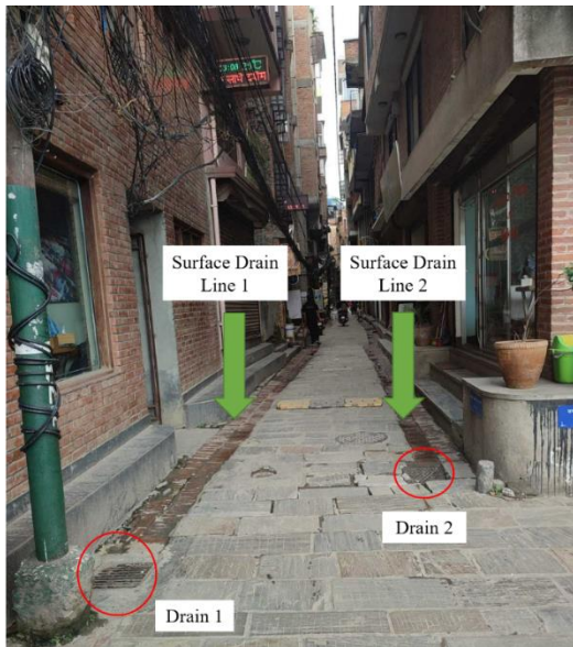
Figure 27:- Drain Lines and Drain
