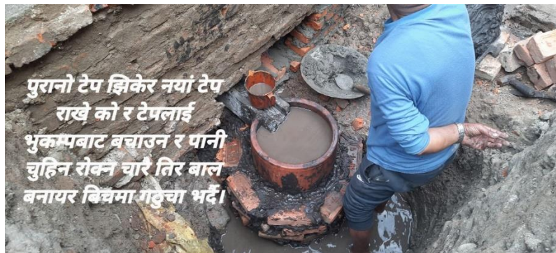
Figure 20:- Hiti Substructure (Tepa)
