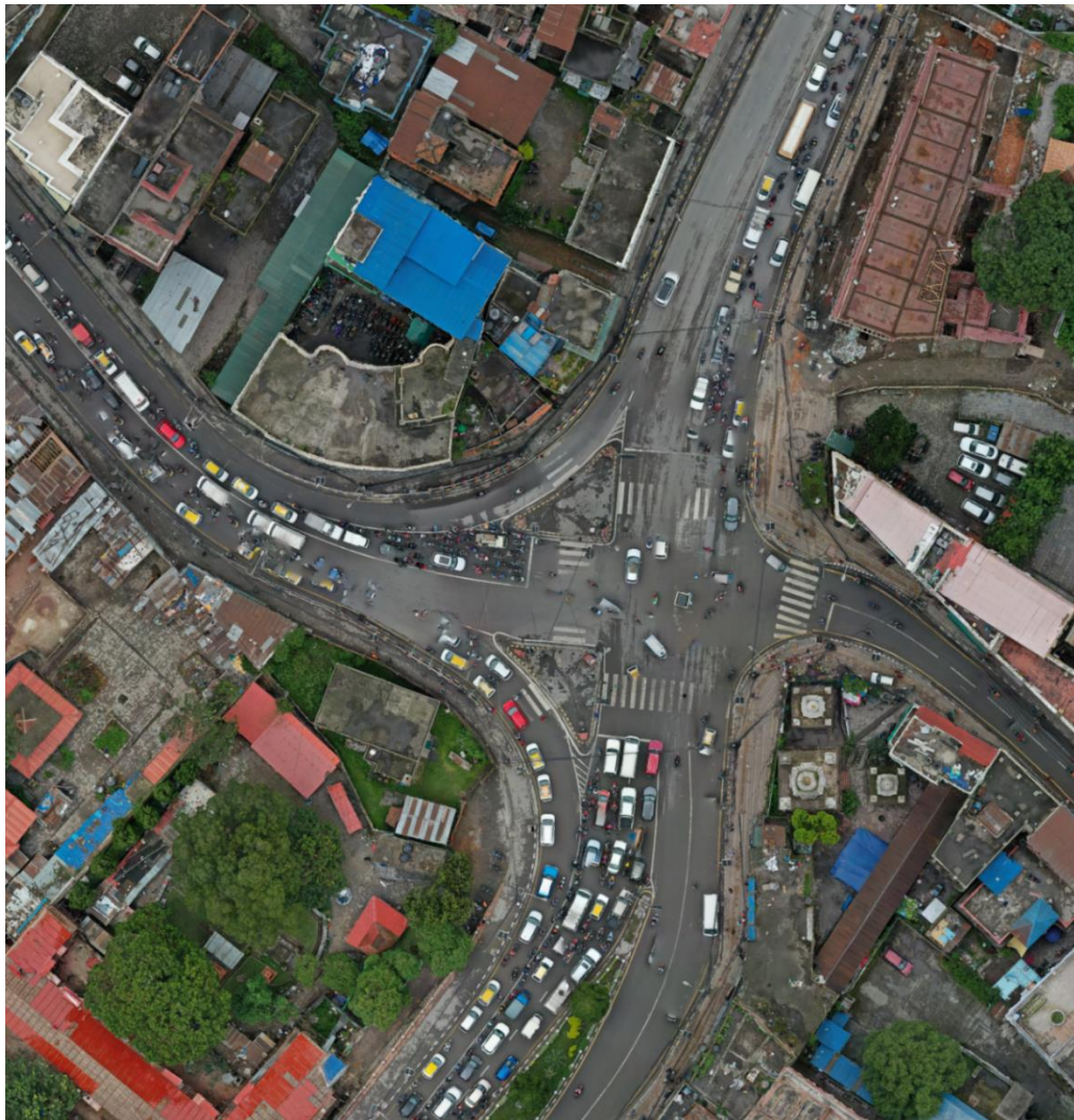
Figure 3-2: Drone Image of Thapathali Intersection
