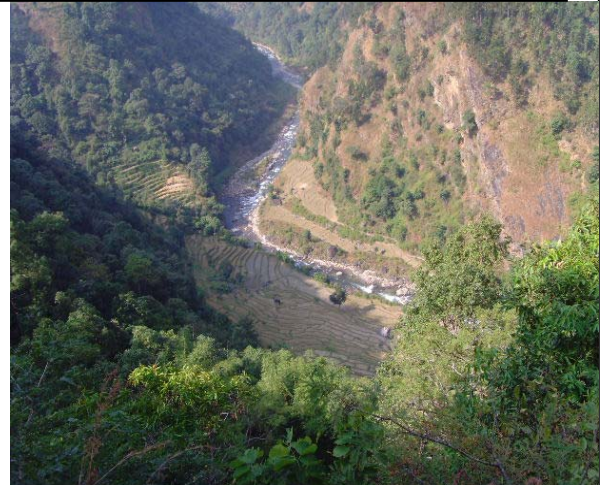
Photo No 4. Proposed Powerhouse site
