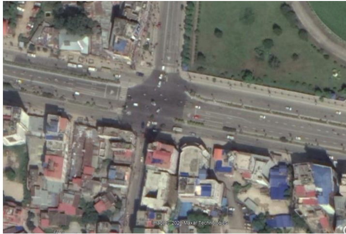
Figure 3 - 2 New Baneshwor intersection
