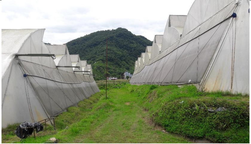
Figure 8. Hi-tech Green House
