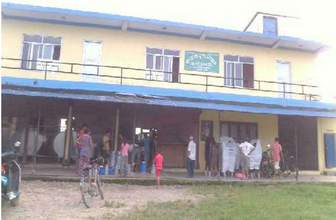
Chilling Center (Panchayan Milk Cooperative Ltd. Pithuwa -7 Madhapur)
