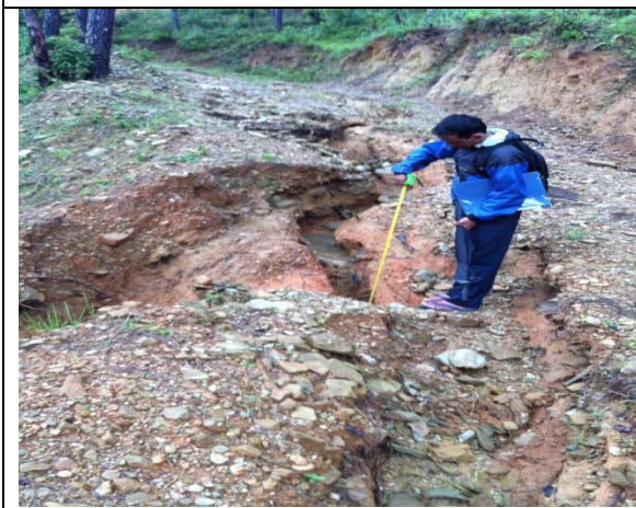
Gully formation in the road surface
