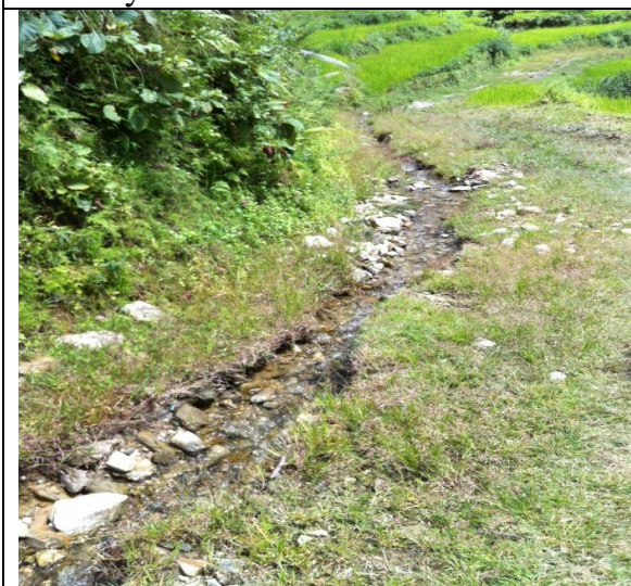
Gully formation in the road surface
