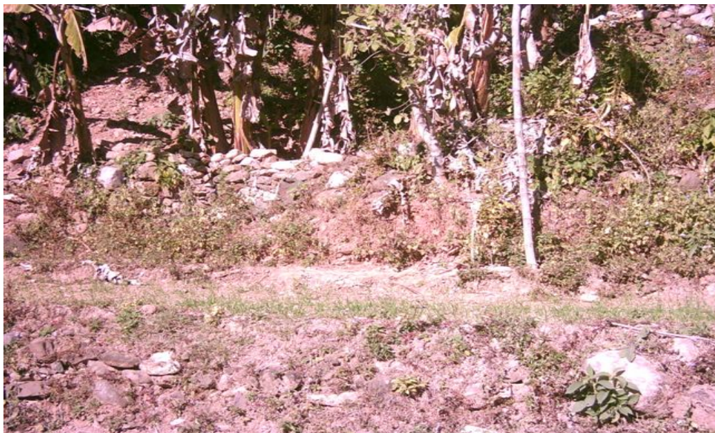
Photograph 2: Gully Protection Work at Ghurmi
