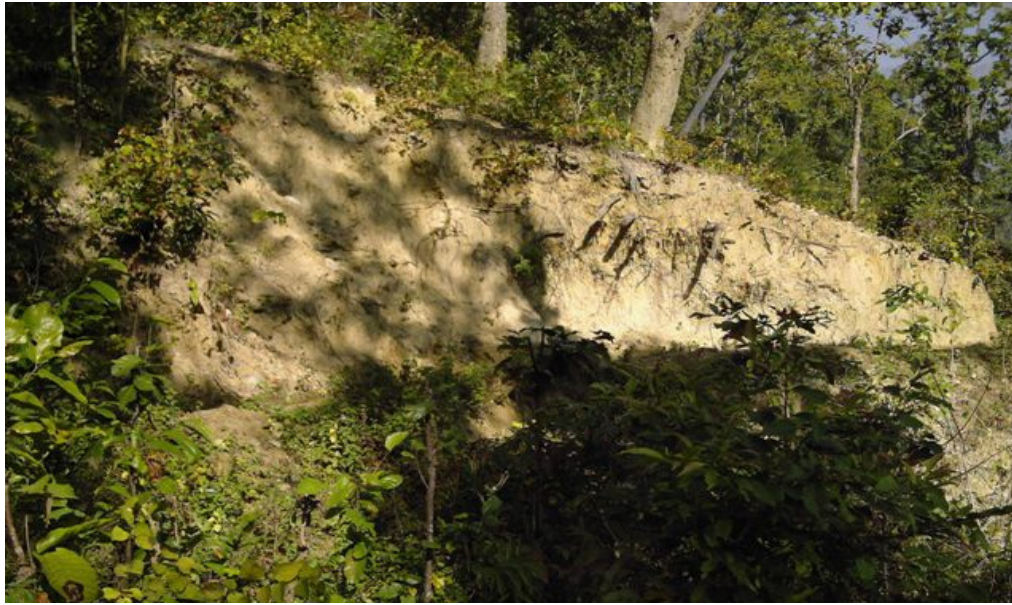
Photograph 2: Gully Protection Work at Bataha
