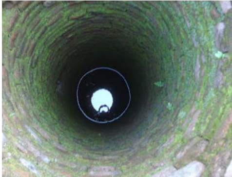
Plate 7 The fig is showing the static water level in a Dugwell at Gaurinj.
