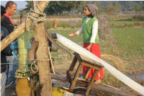
Plate 3: Construction of Shallow Tubewell by Sludge Method at Kesharbag
