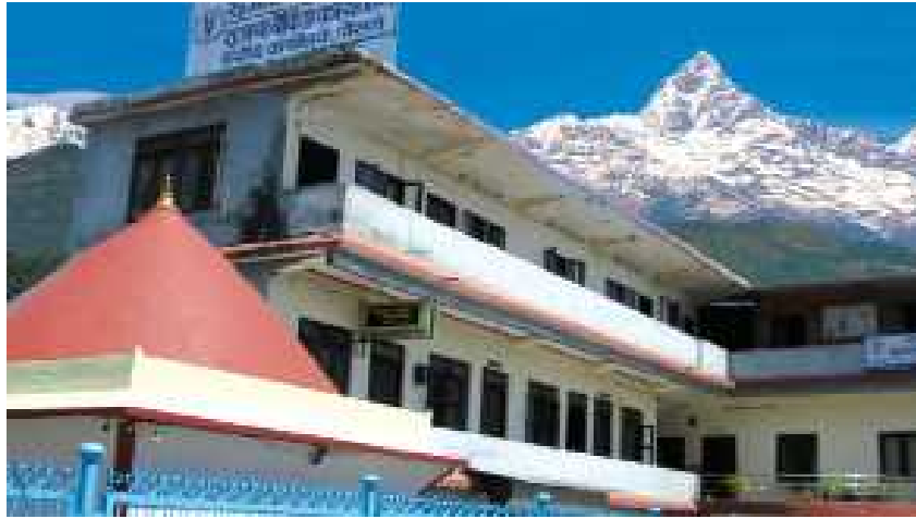
Administrative Building of Sirjana Bikas Kendra.
