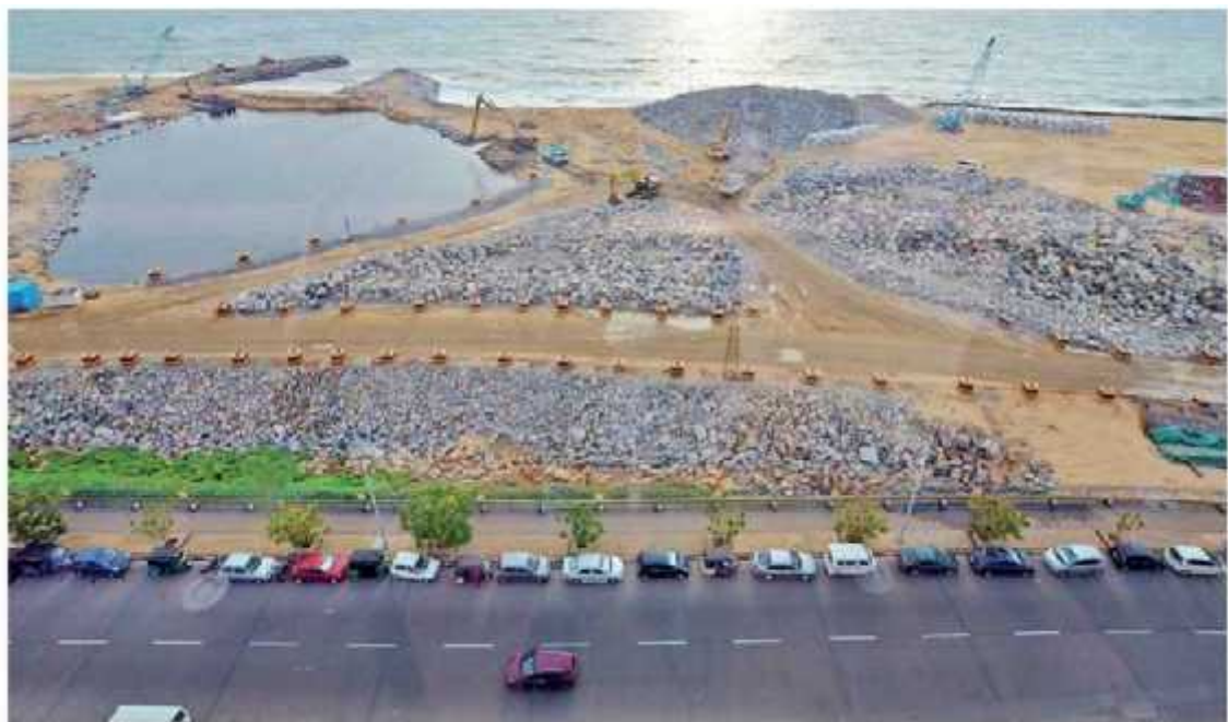
Figure 6.2: View of Colombo Port City (CPC) in 2016
