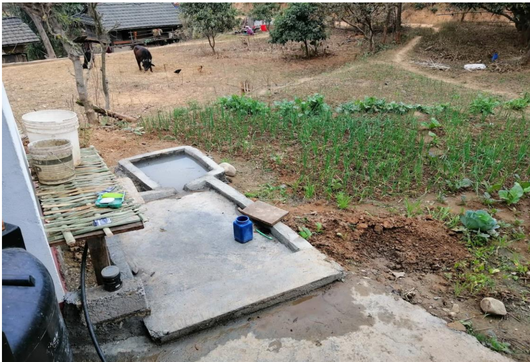
Plate 4: Water collection from kitchen sink by constructing cemented pond as adaptive measures
