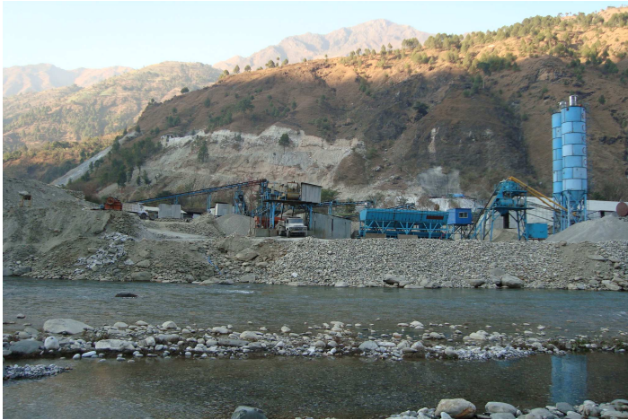
Batching Plant near Chameliya River bank
