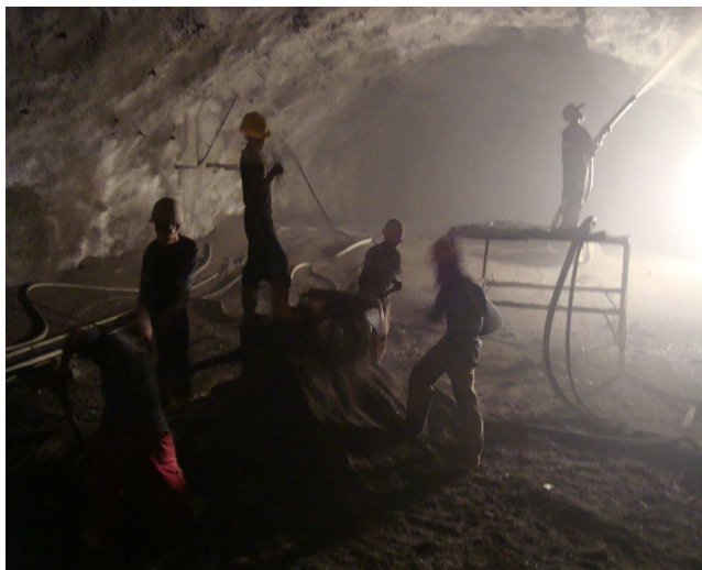
Labor force working inside the tunnel
