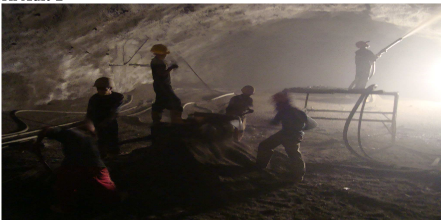
Work force working inside tunnel
