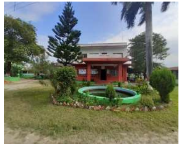
Photo 20: Main office building and Promotion centre
