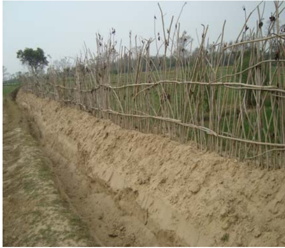
Photo 16. Construction of trench and fence to prevent entry of Blackbuck in field
