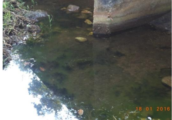
Photo 2. Outlet Channel (S 1 )
