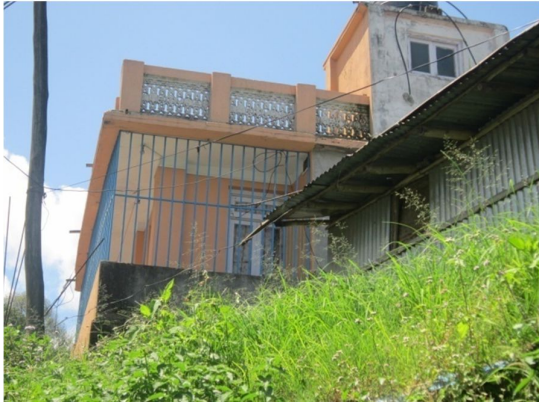
Keeping Fences in house
